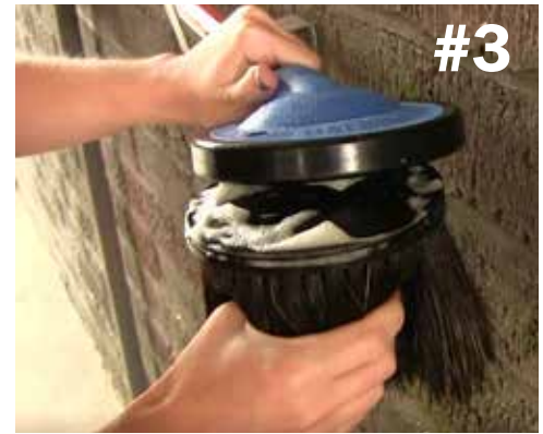
Step 3: Firmly twist the cartridge to the left until you feel it loosen from the threads. Continue twisting while also pulling the cartridge away from the head.
